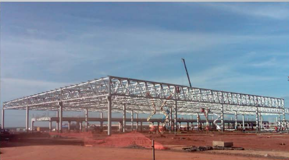
Hyundai Motors - Assembly Shop - 2000 toneladas
